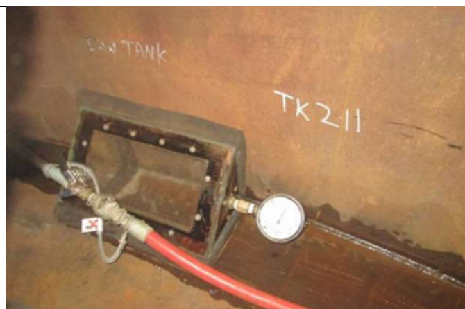
Fonte Vacuum Box Testing (VBT)
