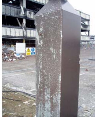
e) Post in car park
