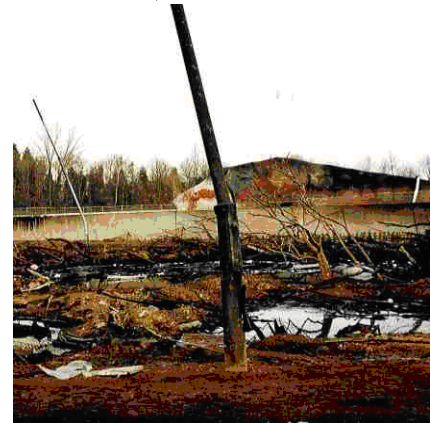
f) Deflected lamp post
